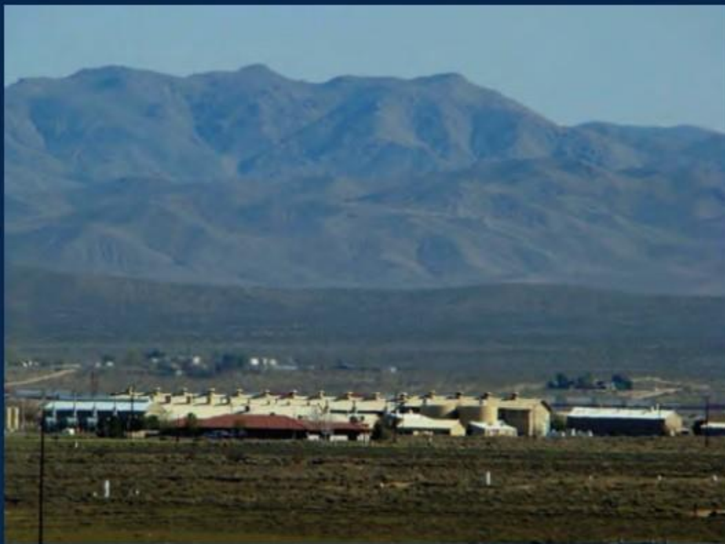
PG&E Hinkley Compressor Station, Hinkley, Calif. (Figure A.1, photo by Steve Perry ARCADIS)
