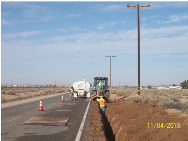
Figure 2: Pipeline Installation Along Santa Fe Road
