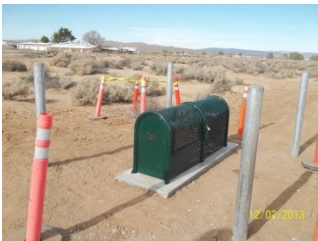
Figure 3: BP at Hinkley School Connection Point
