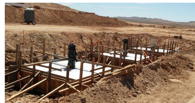
Foundation of Hinkley Road interchange
