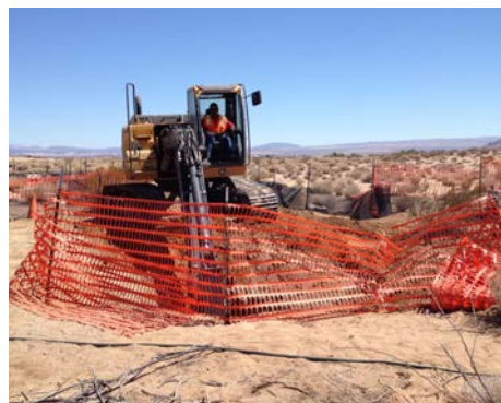
An excavator removes soils and debris.
